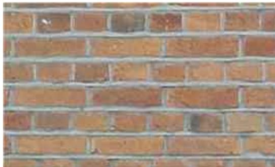
English bond consists of alternating courses of headers and stretchers, with the alternative headers centred over and under the vertical joints of the stretchers.
