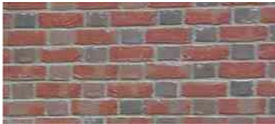
Flemish bond consists of alternating headers and stretchers along each course with the headers centred on the stretchers above and below.
